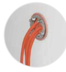
Drilling for cable passage PEXTBALI
